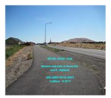
The Keene Road Trail is a 12-foot-wide asphalt path occupying the old Union Pacific right-of-way adjacent to Keene Road. The trail runs between Bellerive Drive and S. Highlands Boulevard.
