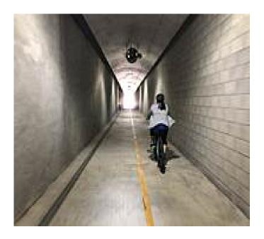
To reconstruct the tunnel, all the wood timbers had to be removed and replaced with steel arches that were then encased in shotcrete embedded with small steel fibers to increase flexibility. The new tunnel will also accommodate the SMART commuter rail line, and the trail will be walled off from the rail line to prevent trail users from accessing the tracks. The trail will have a separate ventilation system from the train track, which will have diesel engines running on the line.
