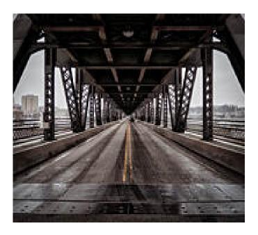
The Government Bridge has two decks: the upper deck has two railway lines, while the lower deck accommodates vehicular traffic, with lanes on each side for pedestrians and cyclists. The deck surface is metal grating.
