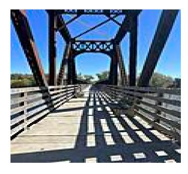
The Montezuma B&O Walking Bridge crosses the Wabash River, connecting Vermillion county and Parke county. Previously an abandoned B&O railroad bridge, the structure underwent a revitalization that included the removal of the old rails and the addition of a new concrete surface and wooden handrails. The new 850-foot-long pedestrian bridge stretches from Water St in Montezuma over the river to Hillsdale, where it meets a paved trail that continues as far as the CSX Rail.
