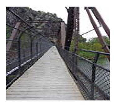
This rail-with-trail bridge crosses the Potomac River near its confluence with the Shenandoah River, at Harpers Ferry, West Virginia. A cantilevered section of the bridge allows pedestrian access between Harpers Ferry and the Chesapeake & Ohio Canal National Historic Park (C&O Canal Towpath) and connects the Appalachian Trail from West Virginia to Maryland.
