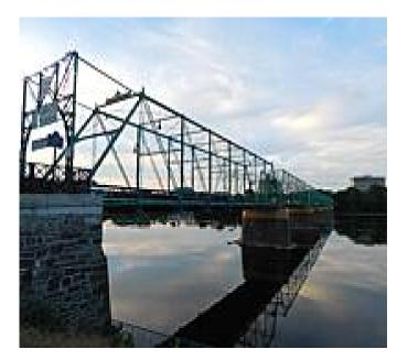
The Calhoun Street Bridge spans 1,274 feet across the Delaware River, connecting Trenton, New Jersey, on its east bank with Morrisville, Pennsylvania, on its west bank. Built in 1884, the intricate iron truss bridge carries motor vehicles on a two-lane roadway and pedestrians/bicyclists in a lane separated from traffic.
